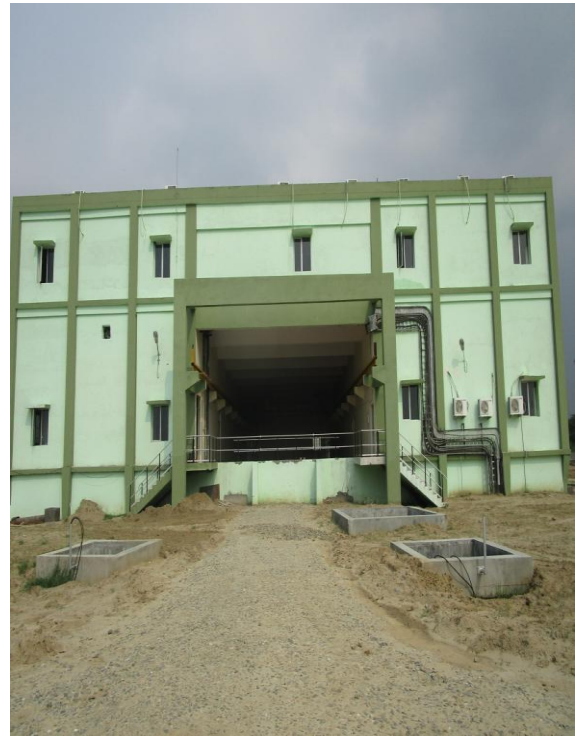
MAIN PUMPING STATION:-
