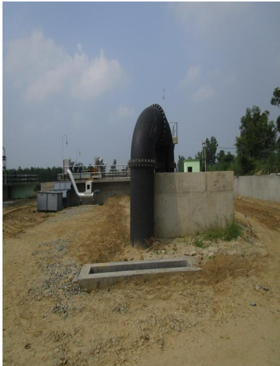
MAIN PUMPING STATION INLET:-
